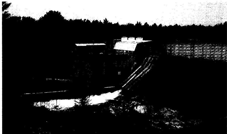
The 2.4-MW Dundee hydro project on the Presumpscot River in Maine is one of five projects featured in a 401 water quality certification case at the U.S. Supreme Court. In the case, project owner S.D. Warren argues that certification is not required because the mere flow of water through a dam does not constitute a discharge into the river.
