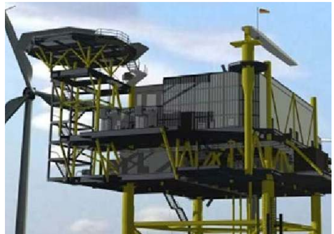
Galloper Offshore Transformer Platform (UK) - Courtesy of Kent
