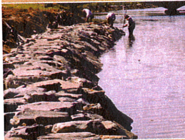
SHORELINE STABILIZATION: CAROLINE COUNTY, MD
