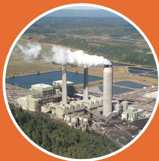
TransAlta Coal-Fired Power Plant
