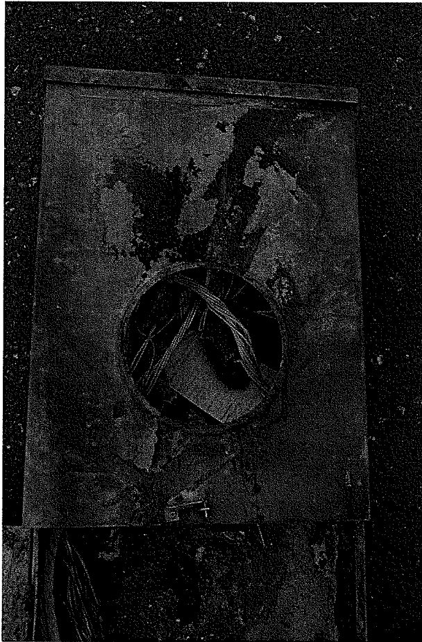
FIGURE 9. A photograph of the Meter Compartment for the subject Meter/Breaker Panel. (Image No.: NEC_1260)
