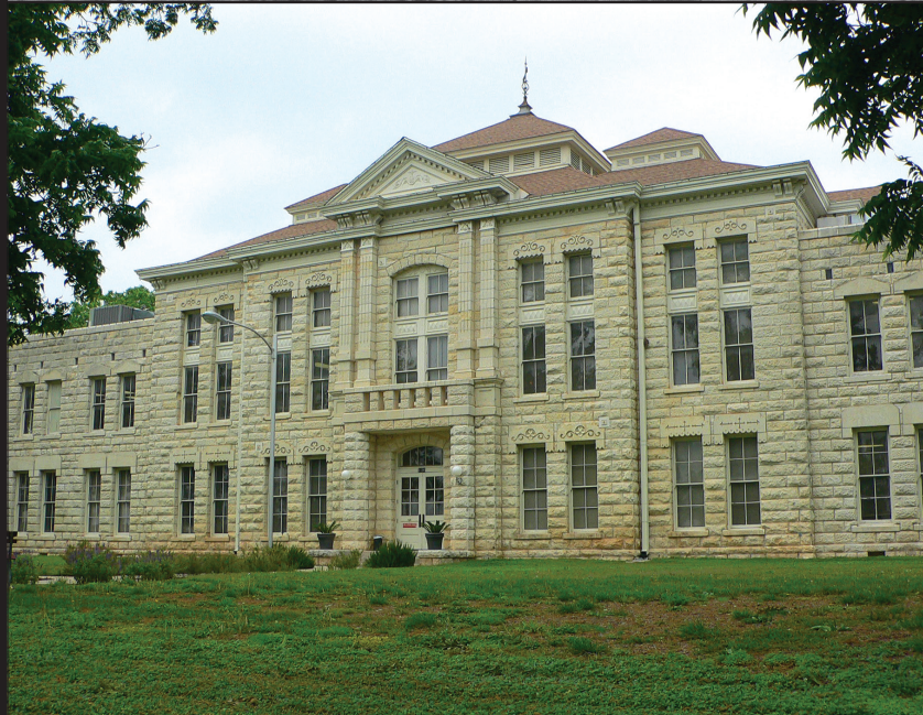
Top: The Medina County Courthouse at the turn of the 20th century. Bottom: The Medina County Courthouse today, with its wings intact.
