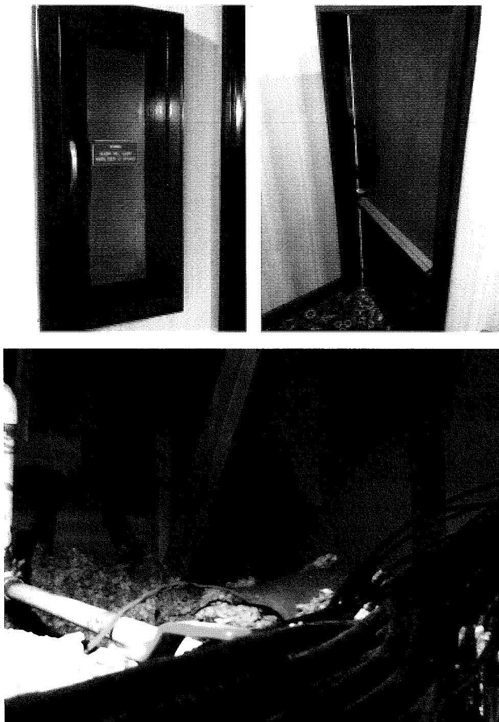
Figure 5. Irregularities noted during the February 20, 2014 inspection of the Country Inn & Suites by Carlson, 4880 University Drive, Huntsville, Alabama 35816. (Top left) Fire extinguisher missing from alarmed cabinet, (Top right) Fire door leading to second floor which does not close properly, and (Bottom) Third floor attic space showing exposed unknown wiring and penetration opening through a firewall or partition in background.
