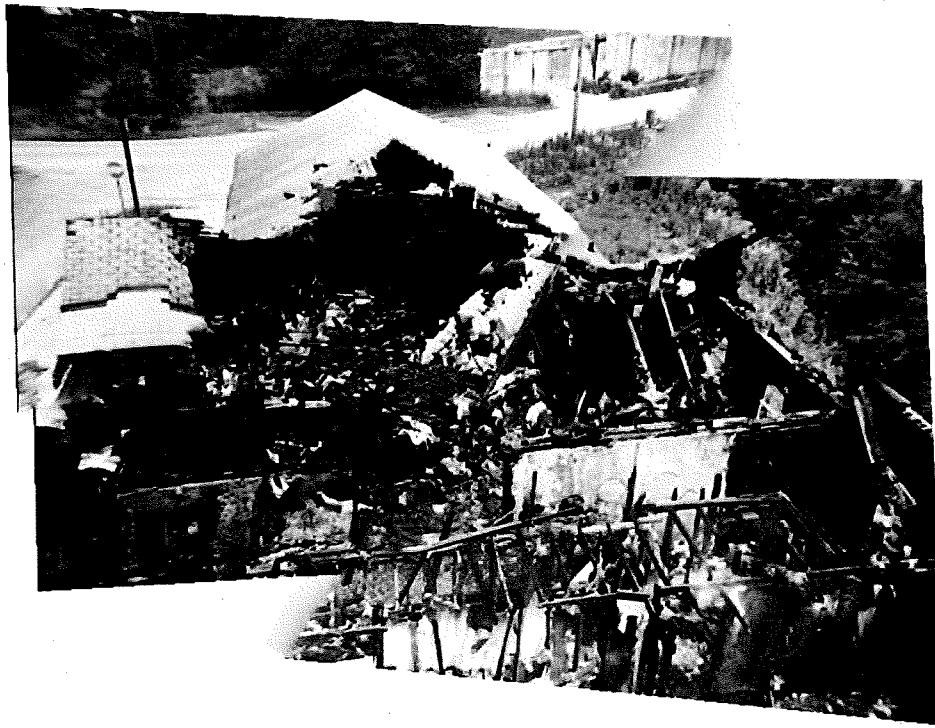
Figure 10. Example showing that the most damaged area is not always the area of fire origin. In this fire test, the origin was at the floor level of the structure in the least damaged area and traveled through the building to the most damaged area in the right foreground.
