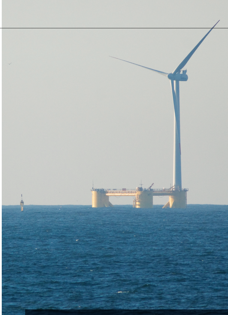
Floating platforms are well-suited for wind farms off the Pacific Coast.
