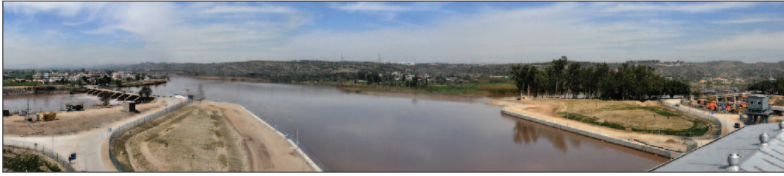
Hydraulic steel works can also be procured as part of an EPC contract, as was the case with the New Bong Escape project in Pakistan. (Image by courtesy of Andy Thick).
